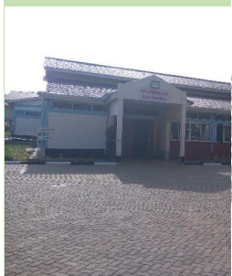
Recently renovated facility hospital Source: OAG Kenya photo
